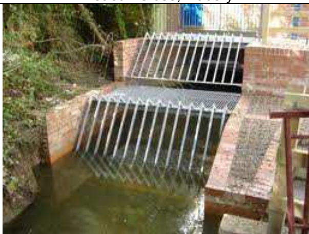
An example of a correctly designed and angled grille
